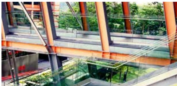
Pinnacle bridge @ Sunway
